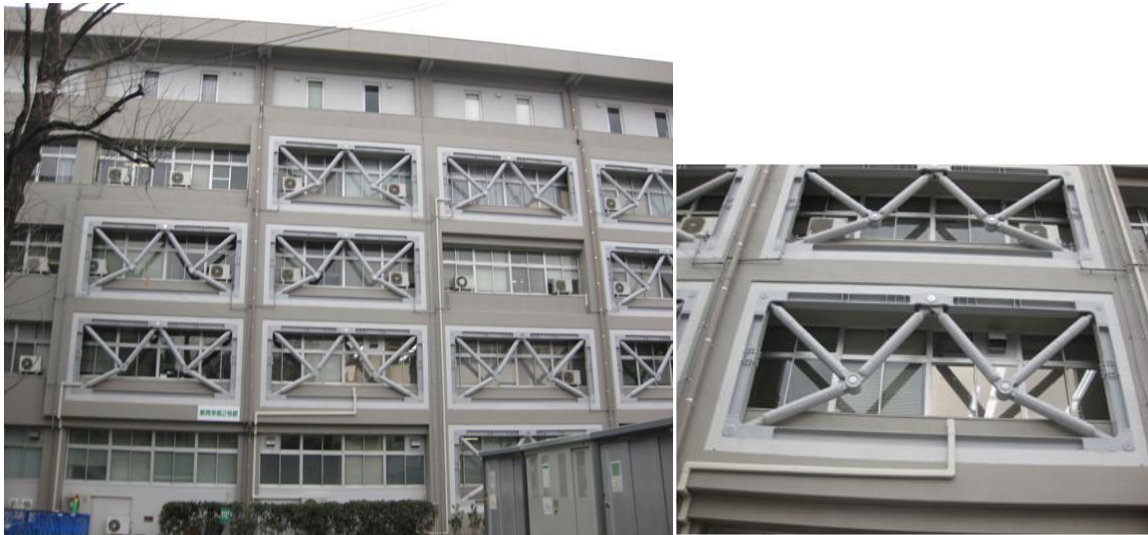
Figure 3-4 Introduction of dampers in existing RCC structure
