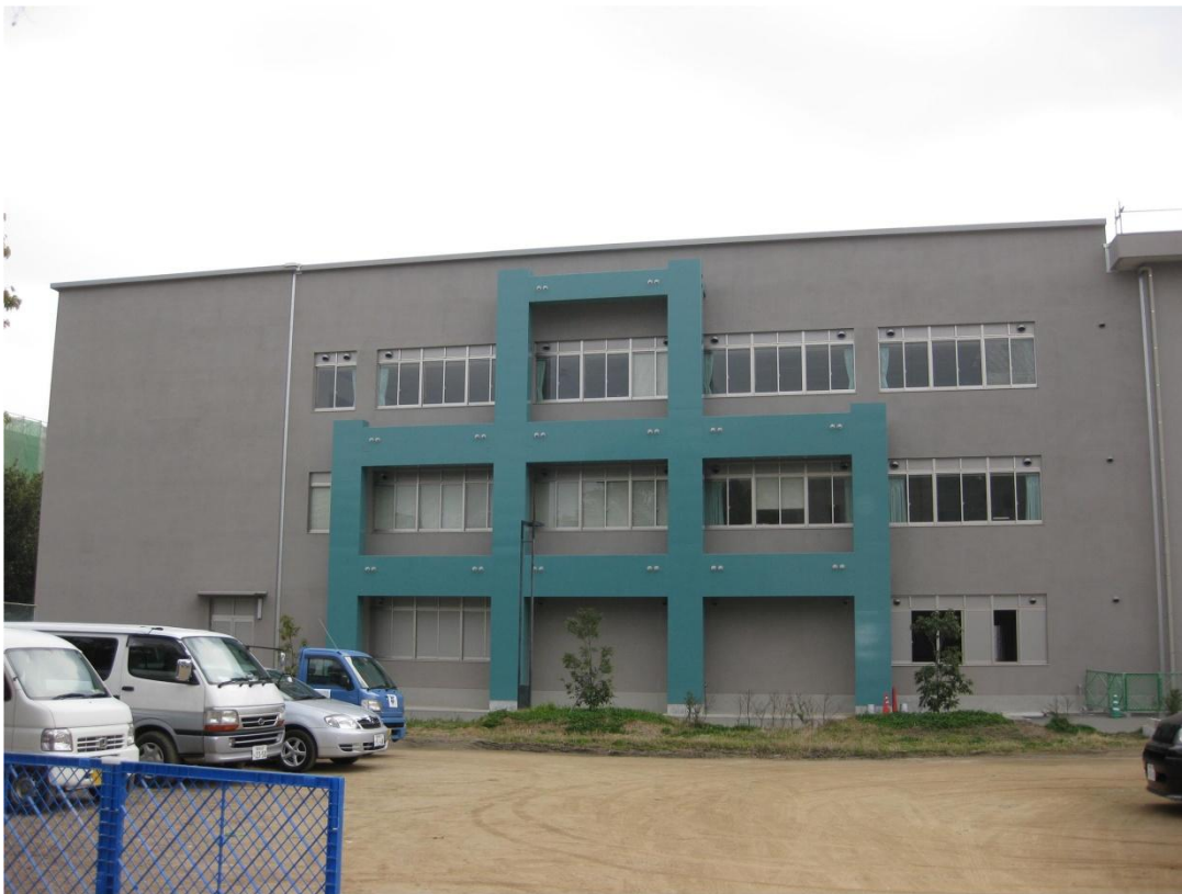
Figure 3-3 Introduction of a steel frame in existing RCC frame building
